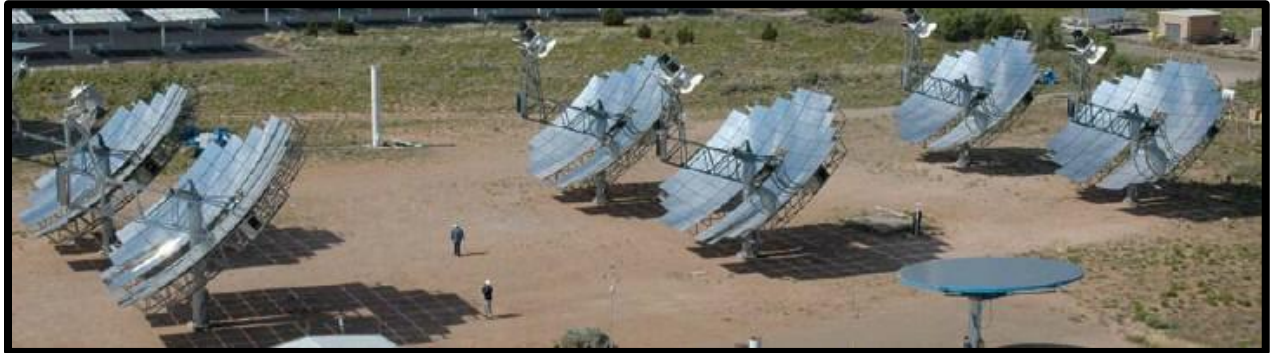
Figure 2: Prototype 150 kW Dish Plant at National Solar Thermal Test Facility (Fraser, 2005)
