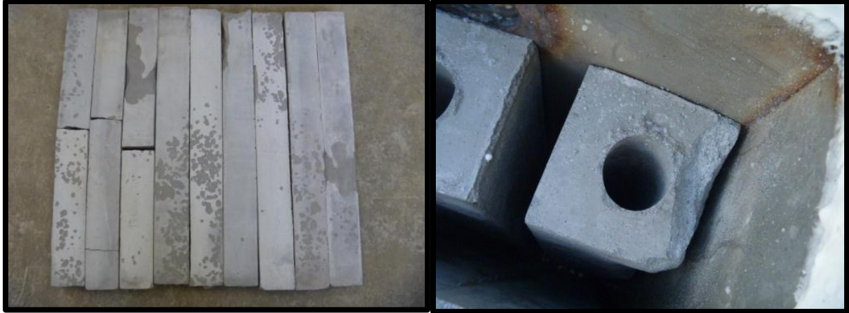
Figure 70: Spalling Damage to TC1000 Concrete Specimens
