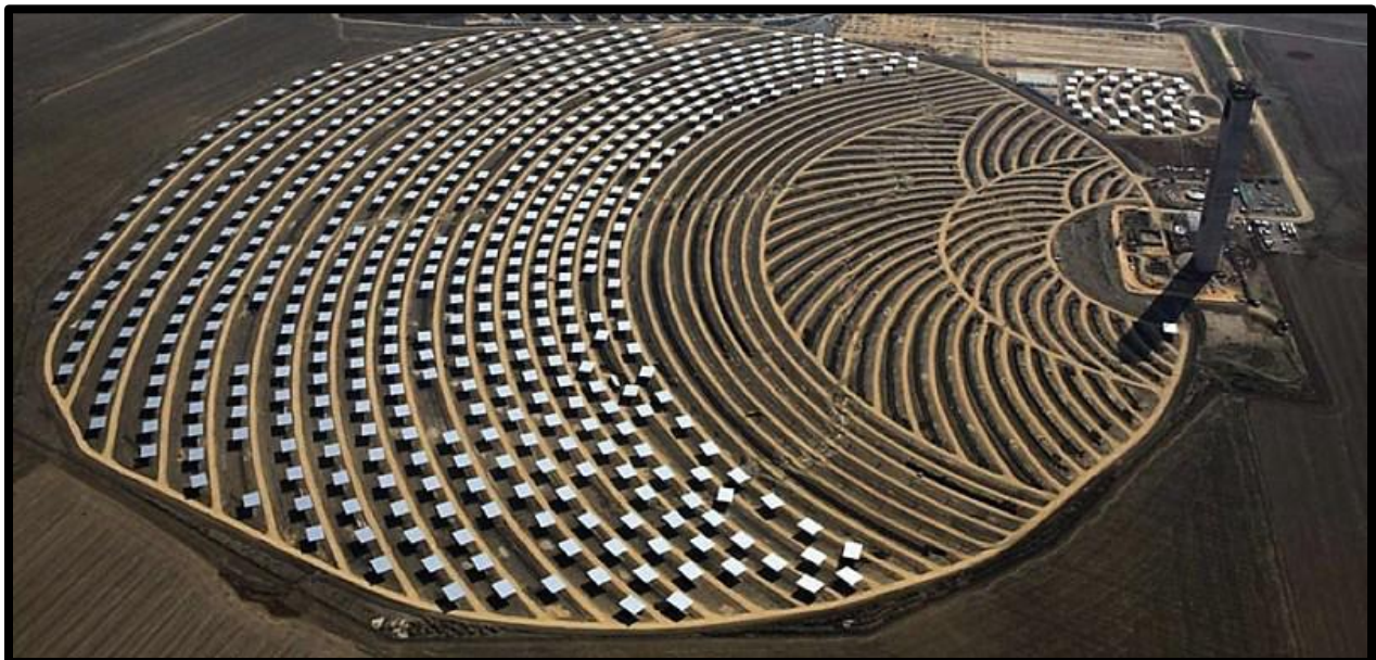
Figure 5: Central Receiver and Heliostats at the 20 MW PS20 Plant in Seville, Spain (Molina, 2009)
