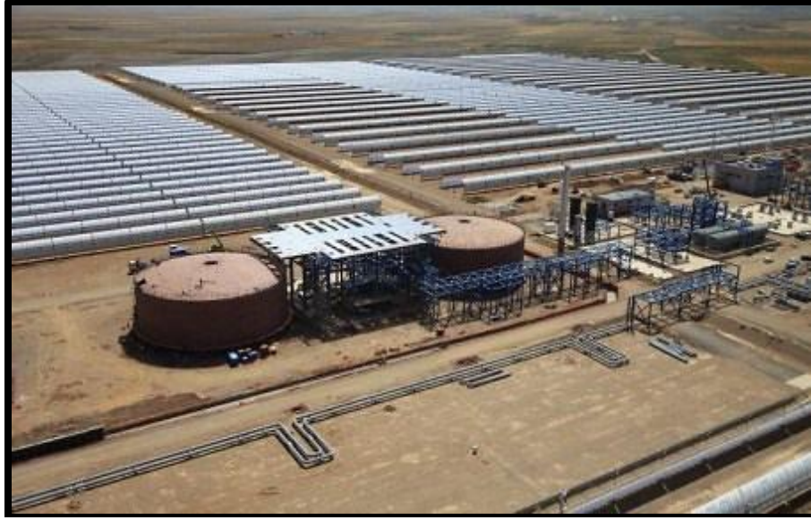
Figure 20: Two-Tank TES and Trough Array at 50 MW Andasol I in Granada, Spain (Craig, 2011)
