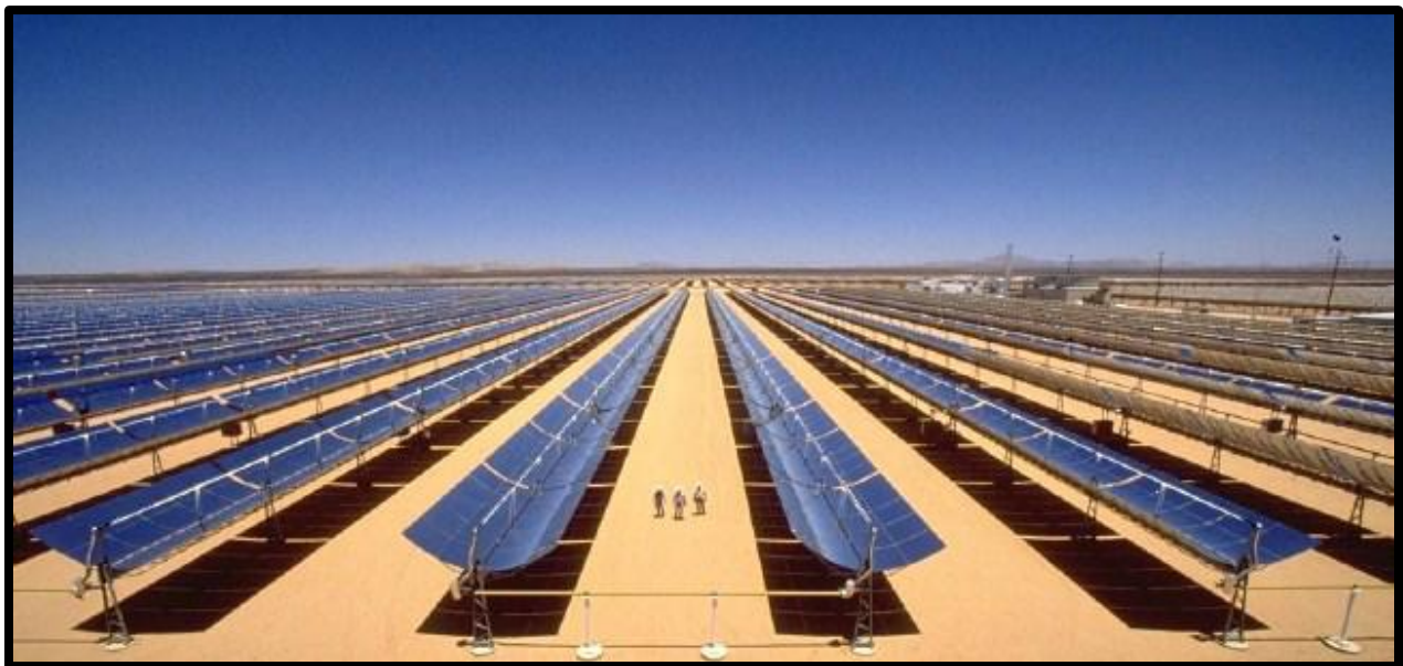
Figure 3: Parabolic Troughs from the 280 MW Power Plant Solana under Construction in Gila Bend, AZ (Siemens, 2009).
