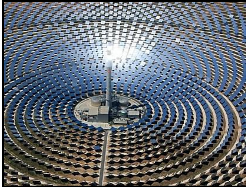
Figure 18: Central Receiver and Energy Storage Tanks at 19.9 MW Gemasolar Plant in Seville, Spain (Harrington, 2012)
