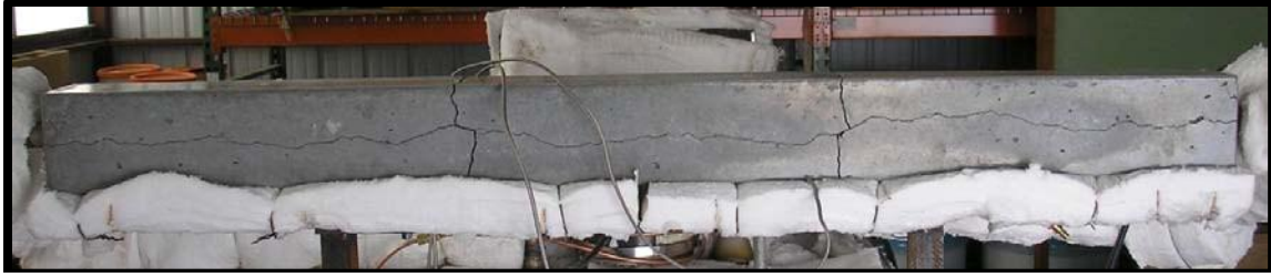
Figure 8: Cracking in Concrete Block with No Soft Material at Interface of Concrete and Stainless Steel Heat Exchanger (Skinner et al., 2011)
