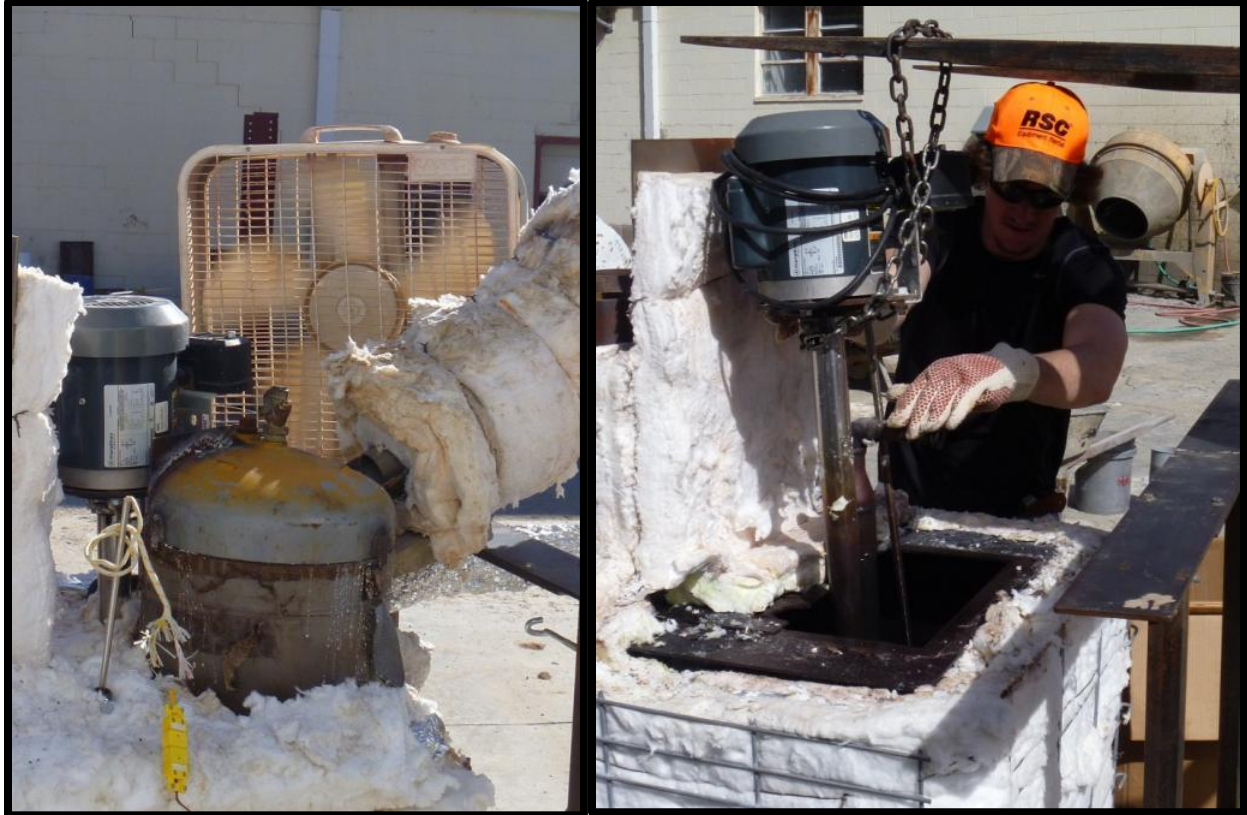
Figure 69: Motor Driving Pumping Unit During Testing (Left) and Pumping Unit Being Removed to Allow Replacement of First Motor (Right)
